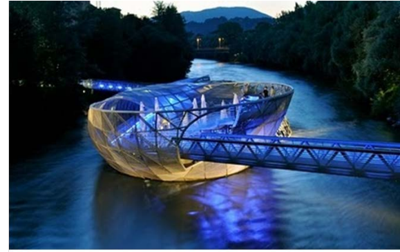
Graz - pedestrian bridge over River Mur. The use of great imagination.
